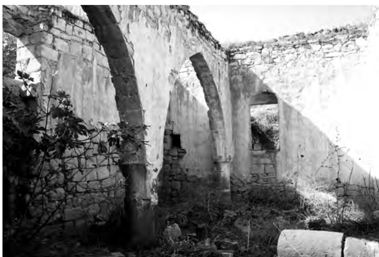
Fig. 3. Interior view of later Ḥibrāṣ mosque. This small, three-aisled mosque is typical of constructions in northern and central Jordan. Like many historical mosques in the region, it had no minaret: a staircase of basalt steps engaged in the exterior face of the qiblah wall led to the roof, from where the muezzin called the faithful to prayer.
