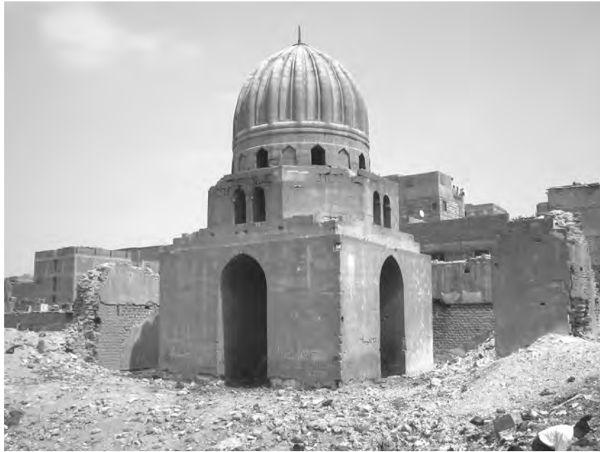
Fig. 7. The dome within the īwān
