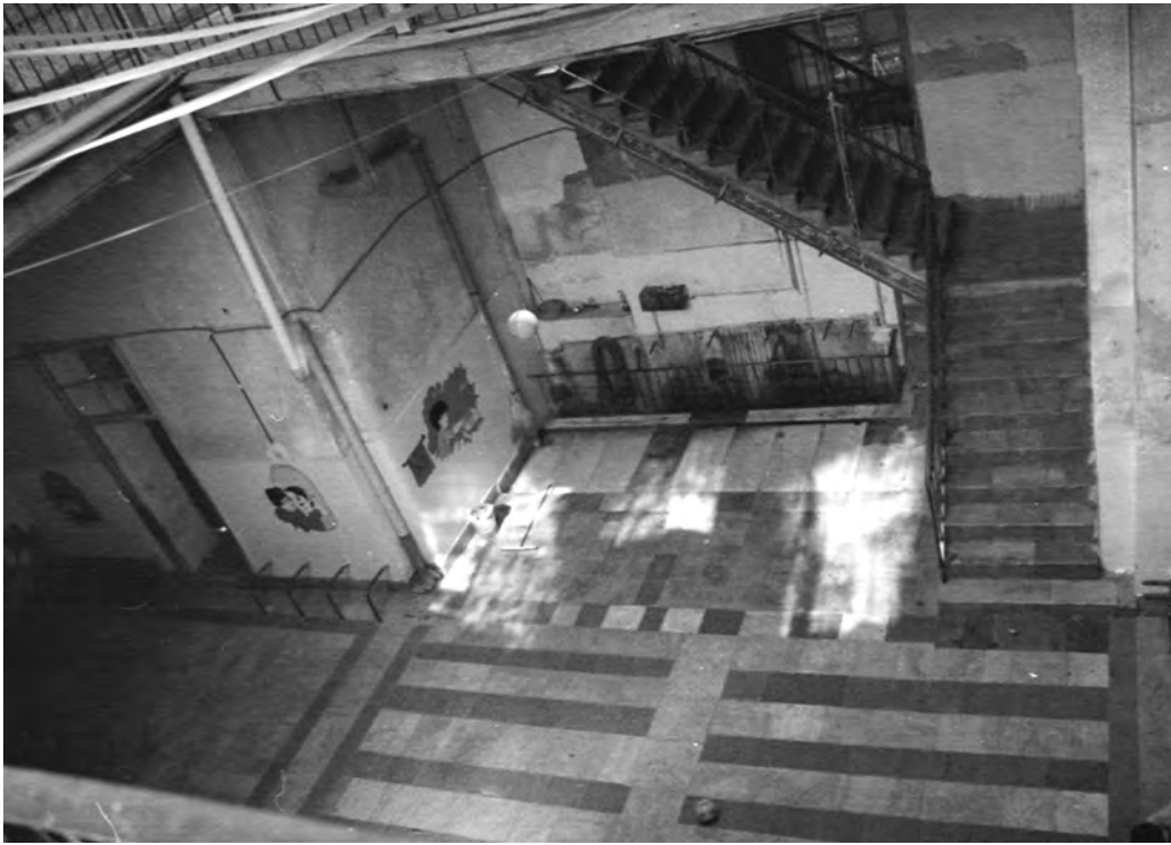
Fig. 11. Damascus, Tankizīyah: interior, view of east īwān
