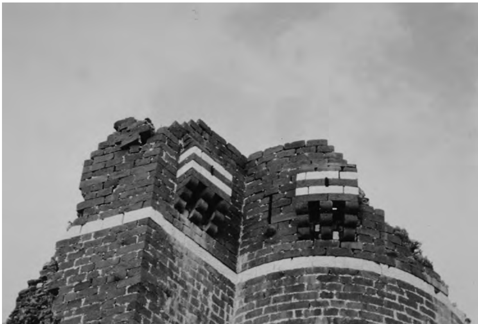
Fig. 10. Marqab castle: Decorative alternation of basalt and limestone courses on the facing of the Mamluk box machicolations
