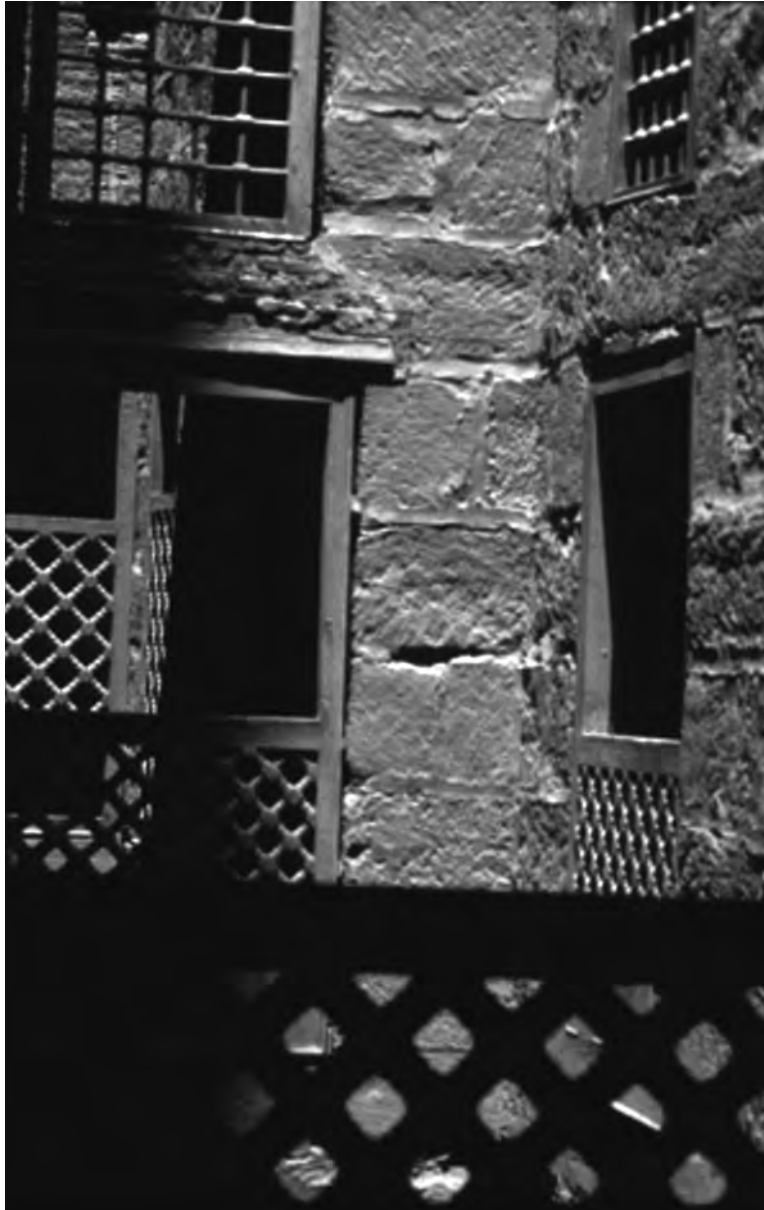
Fig. 24a. Ḥanafīyah Madrasah, Complex of Sultan Ḥasan, Cairo, interior view from living units (H. Al-Harithy)
